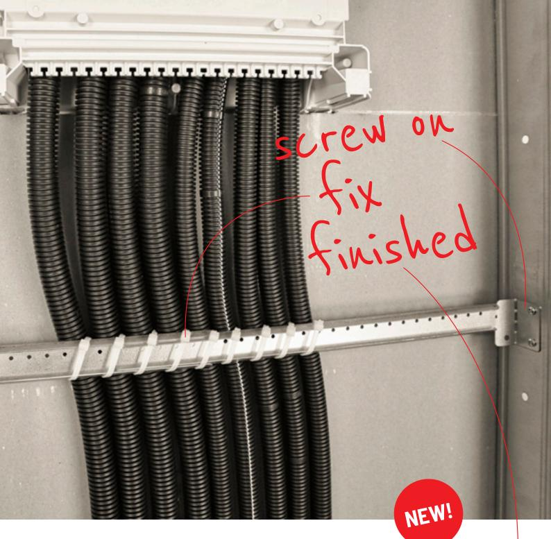
With the telescopic rail TS flexible conduits can easily and quickly be installed in drywalls, e.g. above or below distribution boxes. Find more ideas for quick and easy conduit laying here: **www.schnabl.works**.
