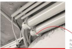
In conjunction with the UVB, the EC Euro-Clip fulfils the requirements of a closed clamp. This prevents the pipes from slipping out.
